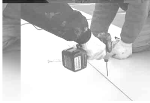
Fix by drilling screw
